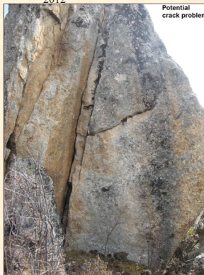
Potential Crack Problem
